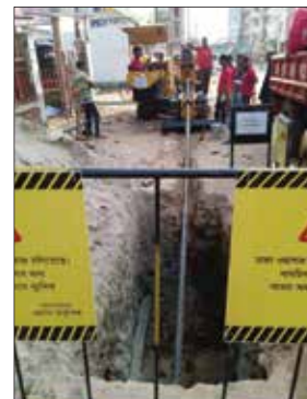
RFL HDPE Pipe used at DWASA ICB 2.7, 2.10, 2.11 Potable water Project
