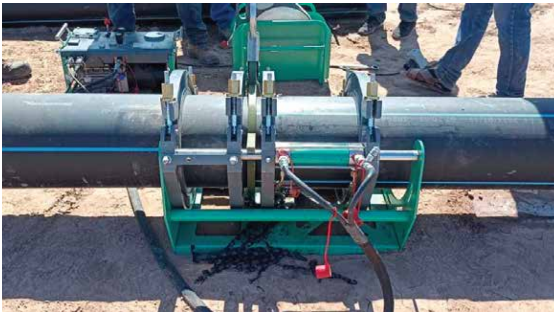
Butt Fusion Welding
