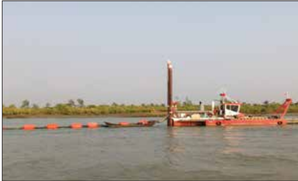
RFL HDPE 800 mm Dredging Pipe at BIWTA Project
