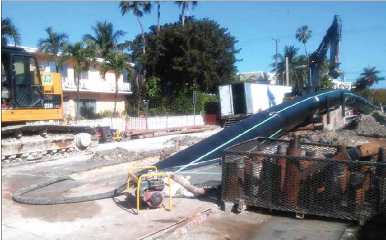
RFL HDPE Pipe Laying
