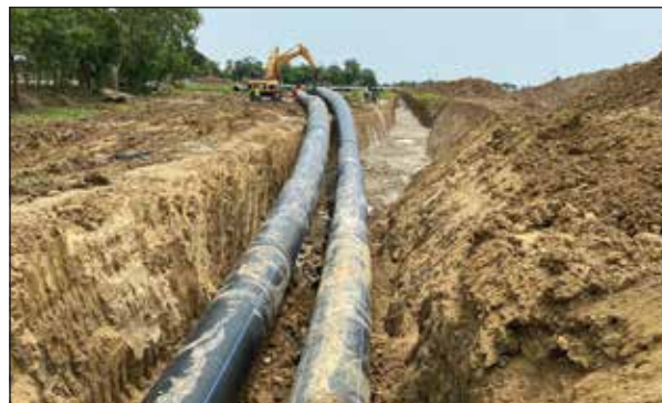
RFL HDPE 1000 mm pipe used in BMDA Godagari,Rajshahi
